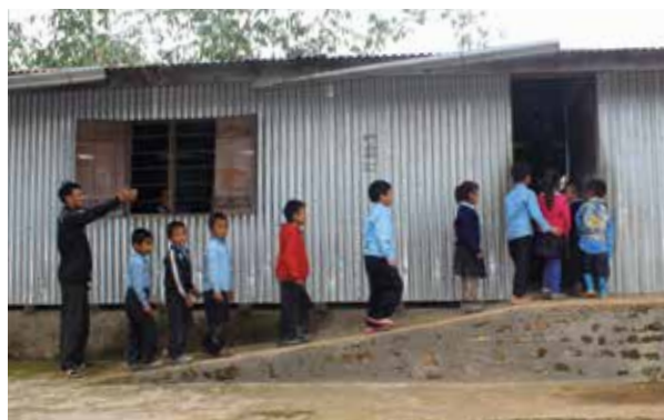
Thirty accessible schools were reconstructed and adapted in 30 villages as well as 15 health centres in 15 villages.
